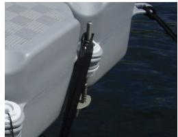
Once the airbag is in place, put the straps on the other side of the Candock dock without tightening the side straps. Also place the center straps by inserting them in the white bolt. Use the front strap of the airbag and the 4 remaining straps to secure the hose along the dock by passing the strap around the pipe and into the white bolts.
